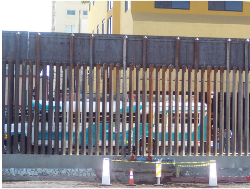
FIGURE 5. New bollard-style wall looking south at the Nogales, Sonora municipal bus station, December 2011.
